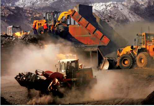
Kohlehalde in Fuxin in Liaoning
