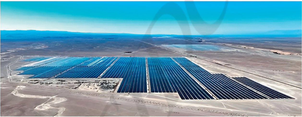
Figure 4-31 CEME1 PV Power Plant in Atacama Desert, Chile
