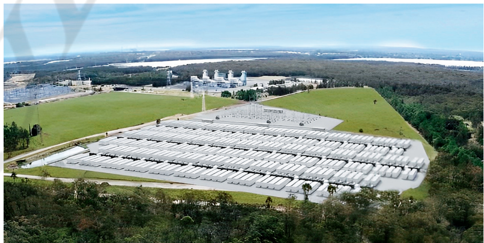
Figure 4-46 Rendering of Waratah Super Battery Energy Storage System in New South Wales
