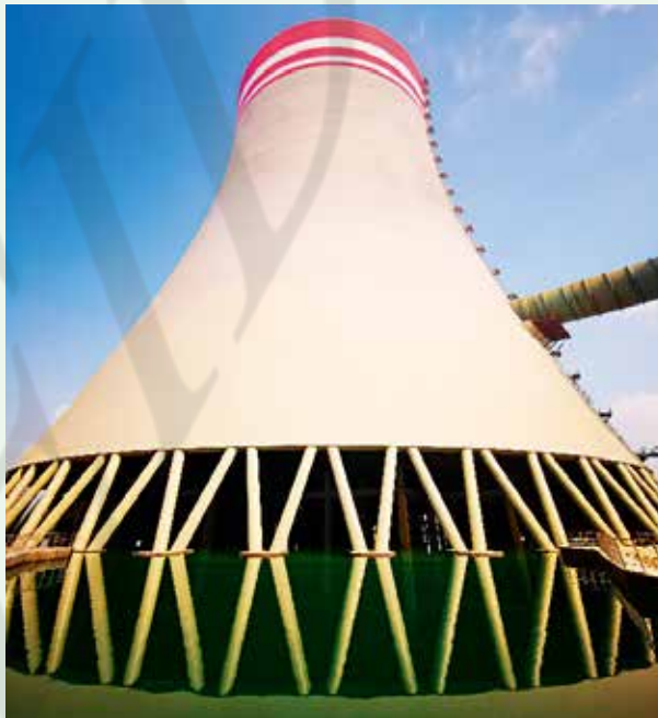
Fig. 1 Smokestack-Cooling Technology at Türkiye's Hunutlu Power Station
