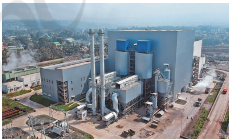
Ethiopia's Reppie Waste-to-Energy Plant
