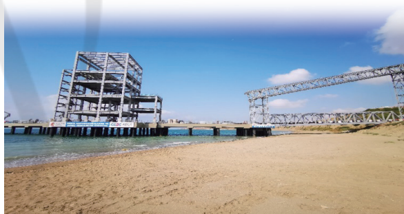
Long-span truss bridge “Turtle Bridge”
