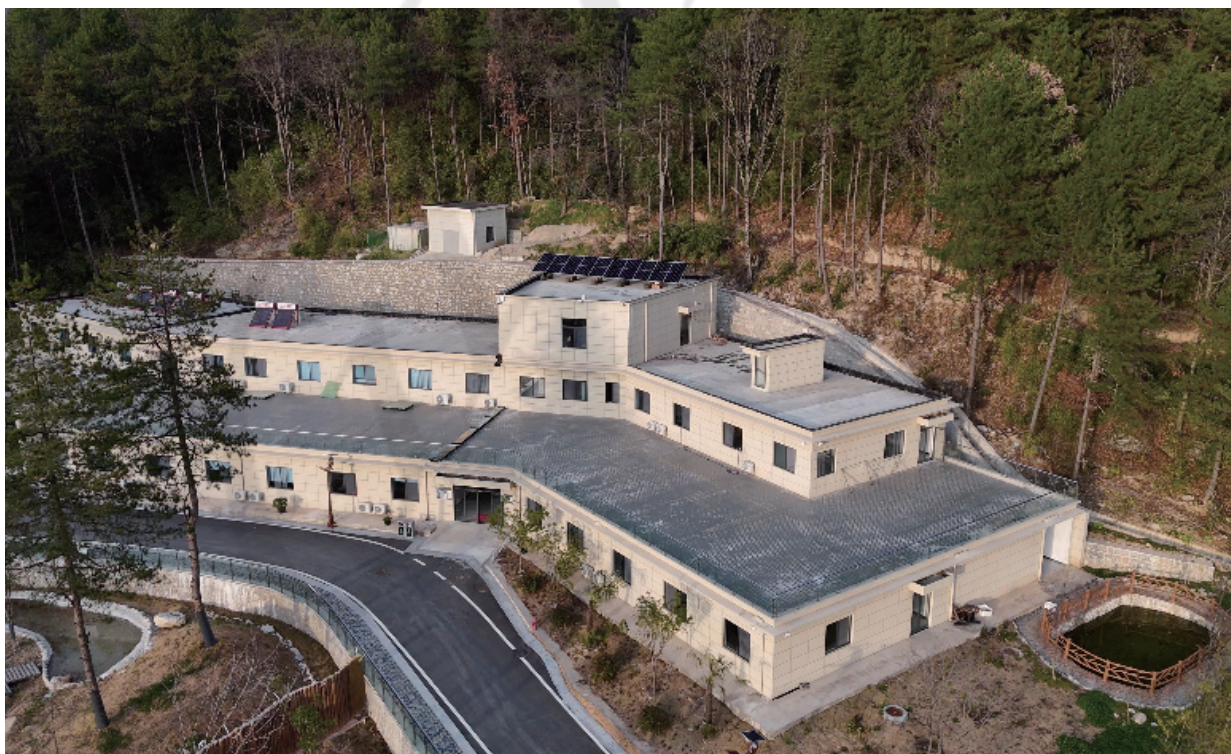
Photovoltaic system at the research building in Qinling Panda Foping Base
