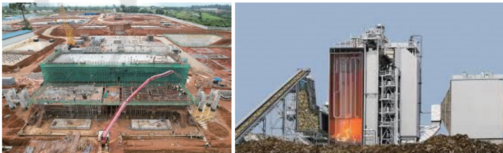
Biomass Power Station Construction Site
