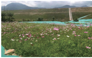
(a) Ecological restoration effect behind the reservoir dam
