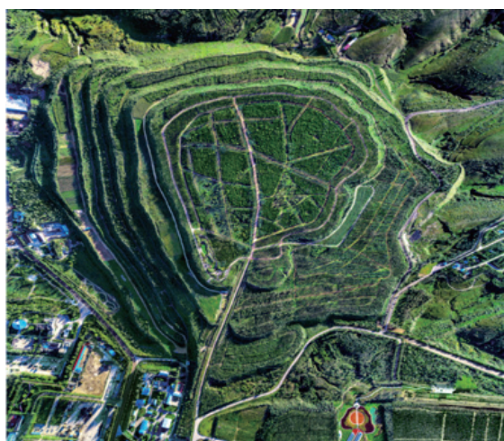
(b) After repair
