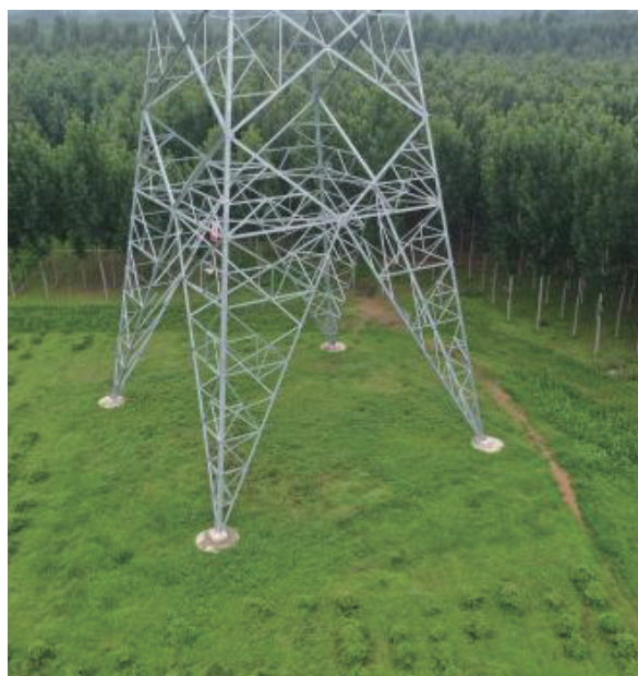
Status of vegetation restoration at the tower site
