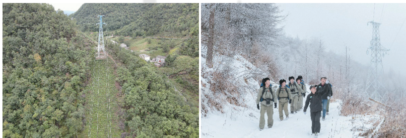
Firebreak belts and power line corridors combined into a dual-channel system
