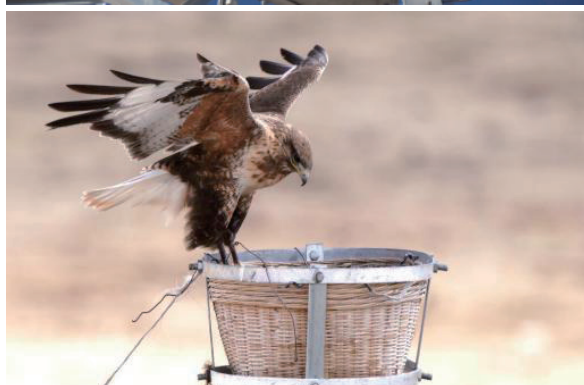
A worker is installing an artificial bird nest on a transmission tower.
