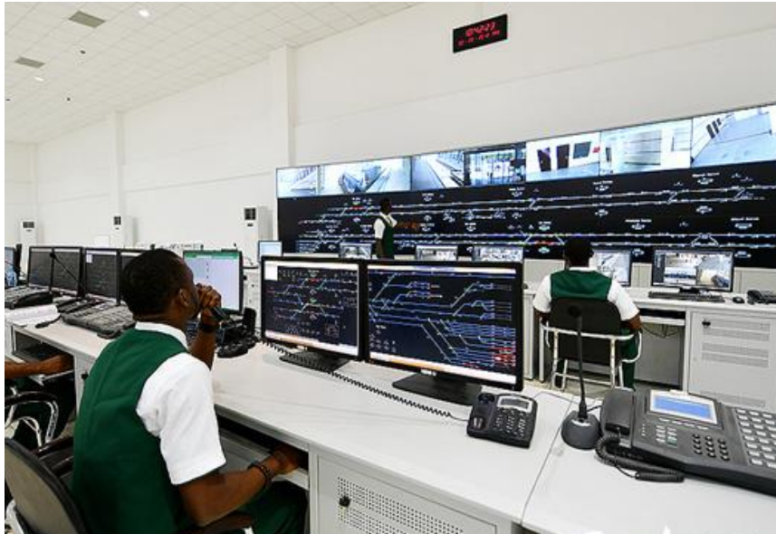
Figure 2.1 ICT Project Integration Center at Luanda New International Airport
