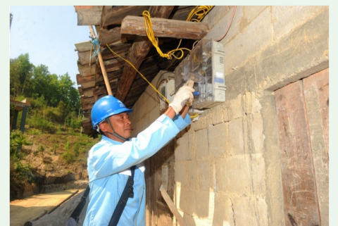
Wei Chenggang checks a transformer outside a villager's house.
